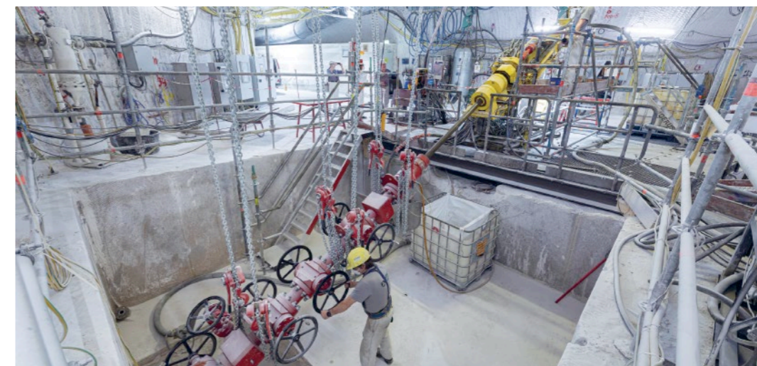
Asse mine: Exploration drilling on the 700 m level for Shaft 5
