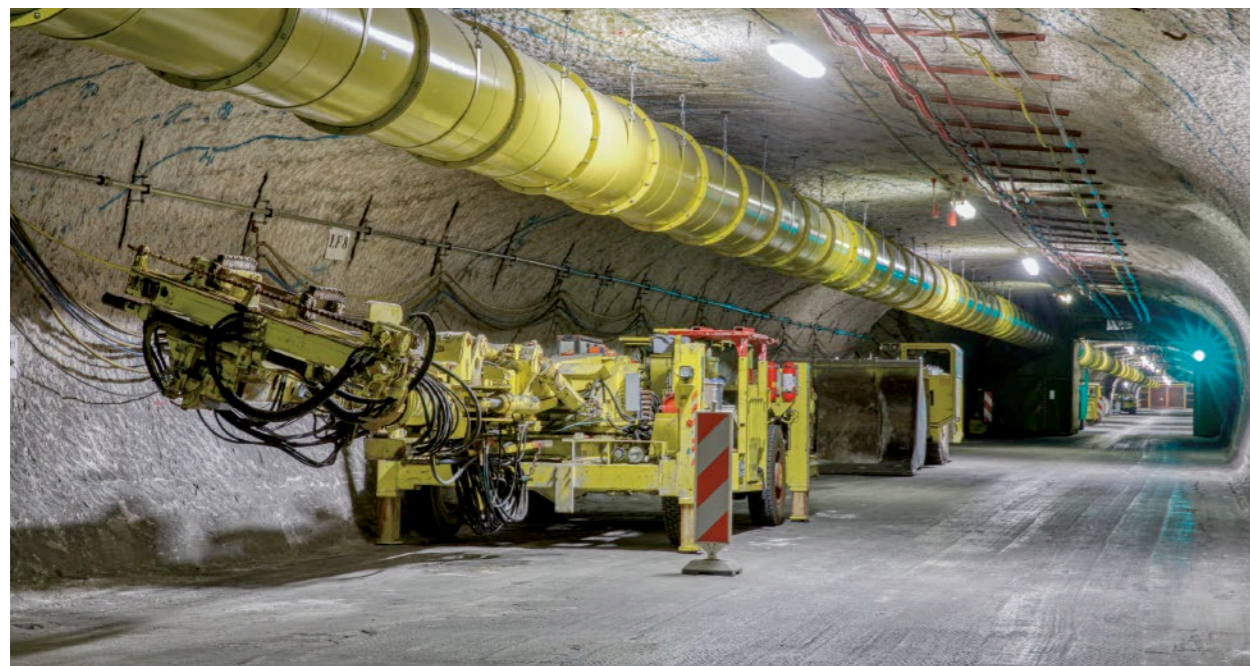
Gorleben mine: Main conveyor section, 840 m level
