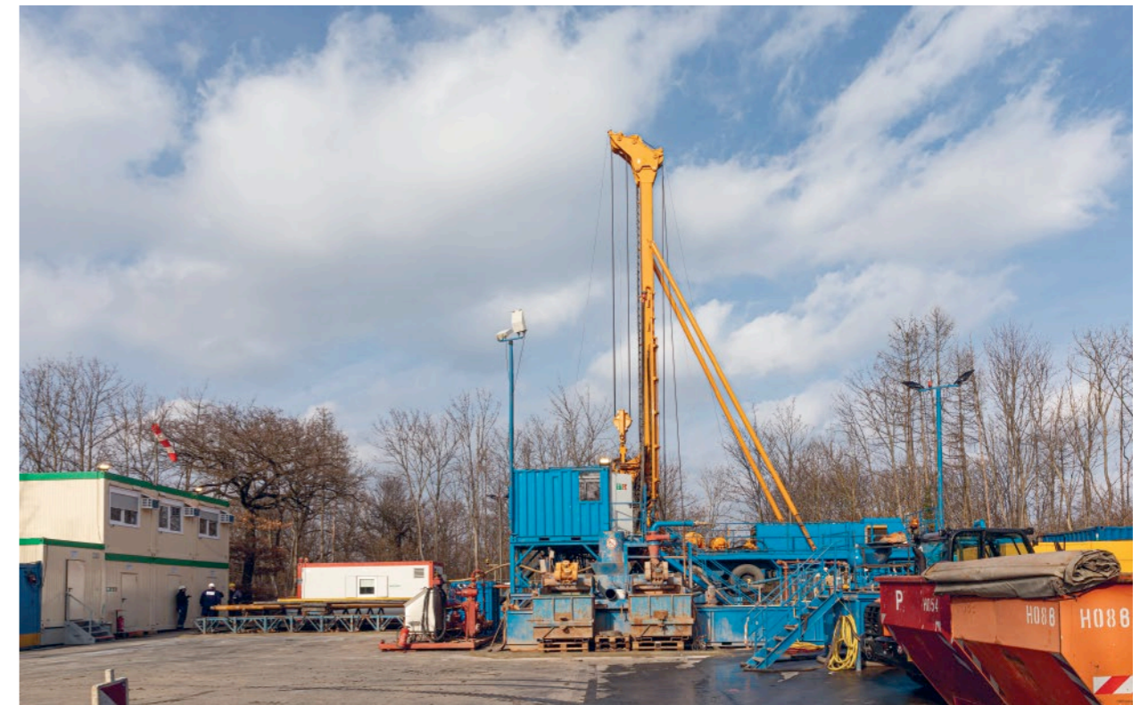
Asse mine: Exploration drilling Remlingen 15
