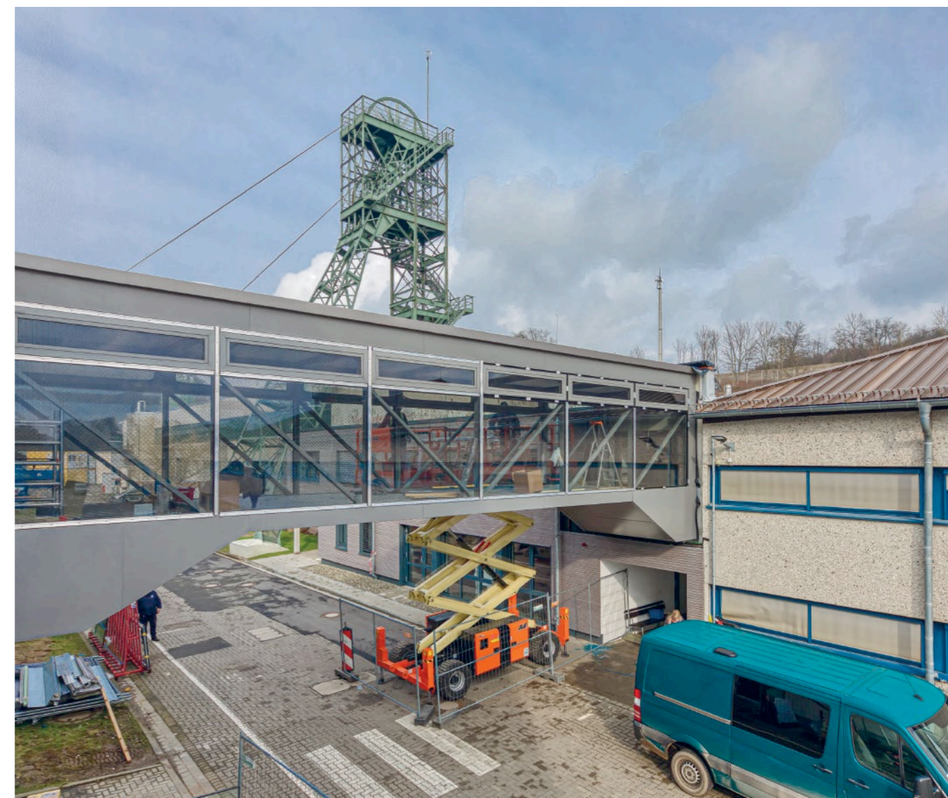
Asse mine: The man-haulage bridge provides draught-free passage from the pithead to the shaft
